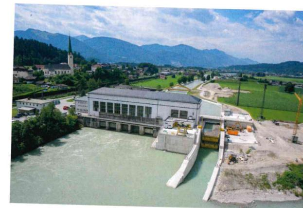
Fig. 5 Kirchbichl Powerhouse and additional weir
