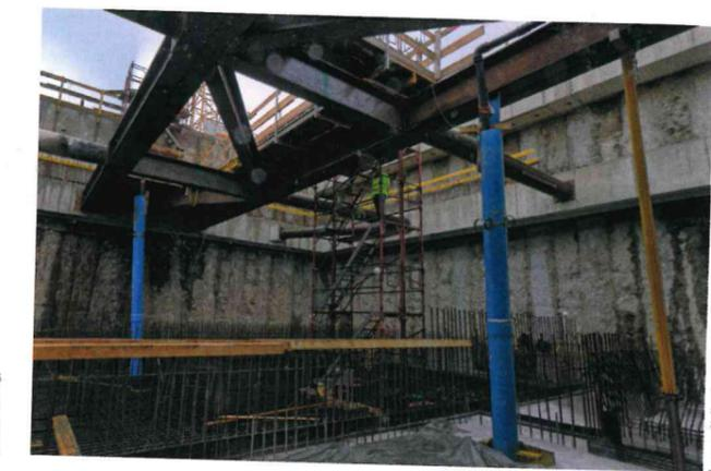
Fig. 6 Finished excavation pit at the weir with bracings
