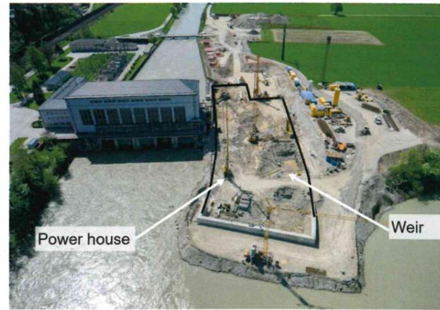
Fig. 7 Kirchbichl Powerhouse and additional weir, starting of foundation engineering works
